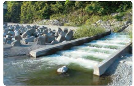
Fishway that was constructed in Toshima Dam
